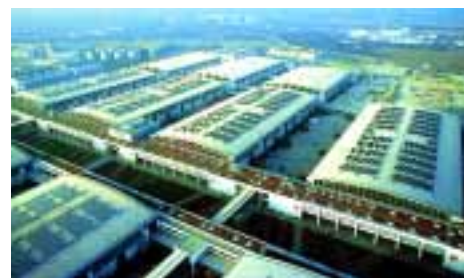
Shell Solar supplies additional power for the Munich Trade Fair Centre, Germany.
