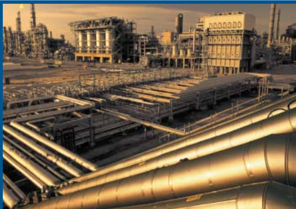
Shell Middle Distillate Synthesis plant Bintulu, Malaysia.
